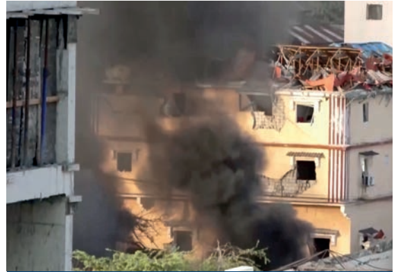
Smoke rises from a National Intelligence and Security Agency (NISA) building following an attack by al-Shabaab, Mogadishu, Somalia, Oct. 4, 2025.
